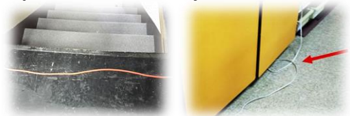
Trip Hazards Caused By Electrical Cords
